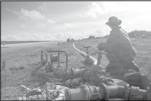
Marine Corps Lance Cpl. Antonio Sanchez, an expeditionary fuels technician assigned to Marine Wing Support Squadron 171, Marine Aircraft Group 12, 1st Marine Aircraft Wing, conducts a pressure test on fuel hoses during an Aviation Training Relocation program at Tinian, Northern Mariana Islands, Jan. 17. The squadron enables expeditionary aviation operations by establishing forward arming and refueling points in austere environments across the Indo-Pacific region. U. S. Marine Corps photo by Lance Cpl. David Getz
